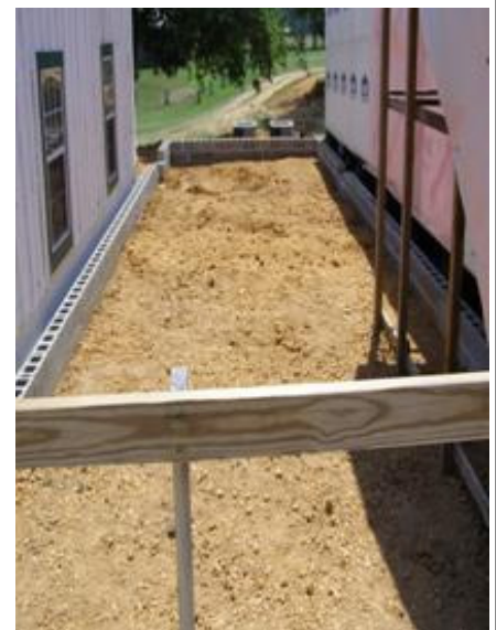
Our finished foundation
